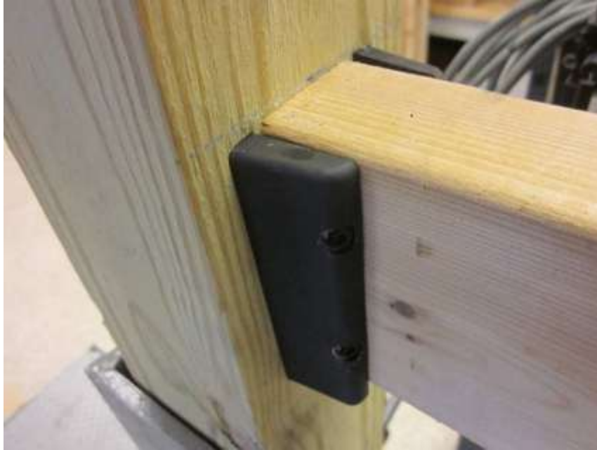
Photo No. 5 Nylon Rail Bracket Installed
