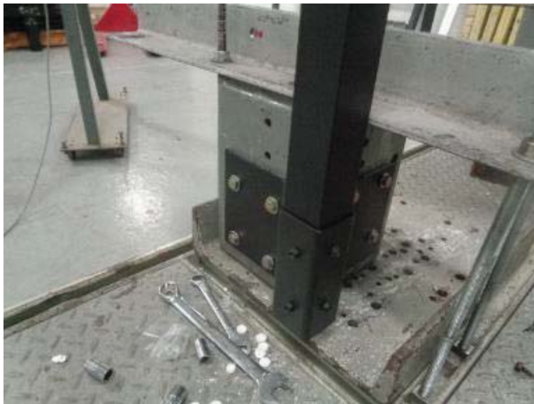
Photo No. 2 Outside Corner Bracket Attachment
